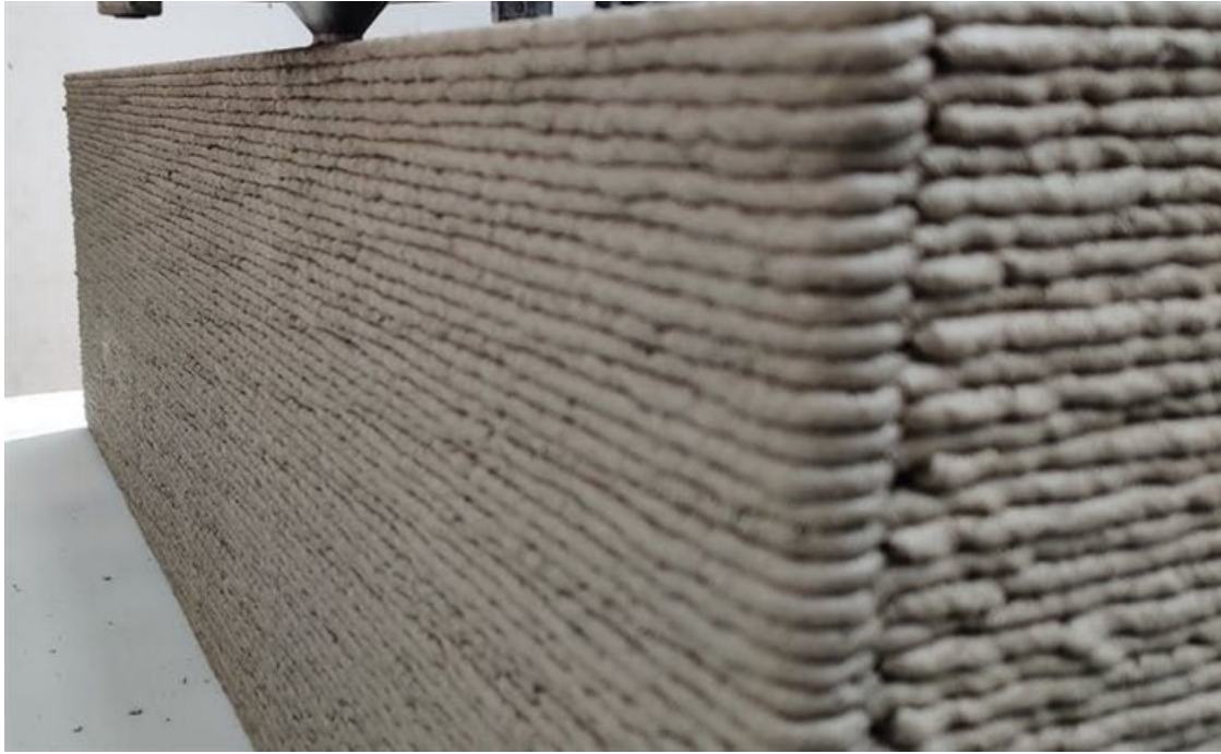
3D printed layers of a wall element. Mehdi Chougan, Author provided
